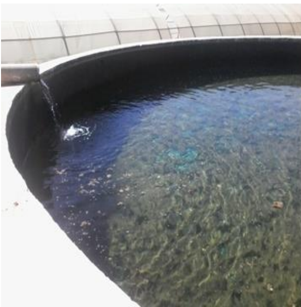
Photo 4. Water storage basin
