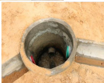
Photo. 2. Water distribution by buried pipeline
